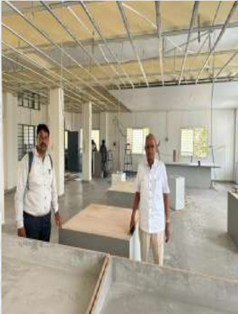
Construction & Interiors for CD Printing Laboratory
